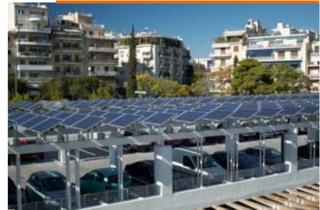
GARAGE MOUNTED PV AT U.S. EMBASSY ATHENS
