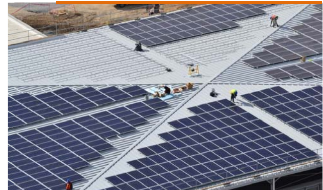
ROOF MOUNTED PV AT U.S. EMBASSY MONTERREY
